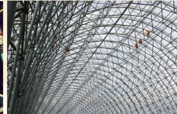
网架拼接 Grate structure assembly and fixing
