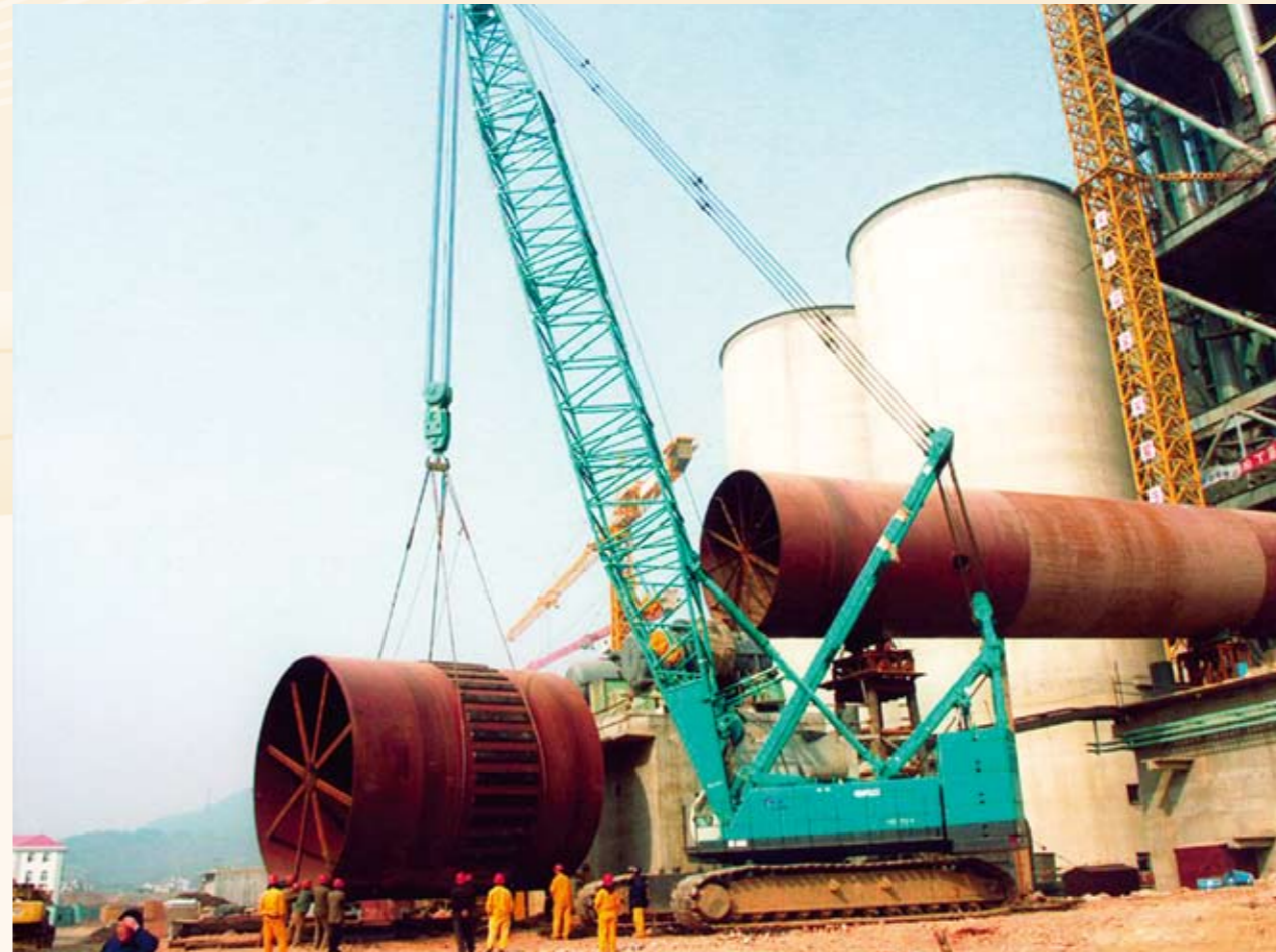
设备安装 Equipment installation
