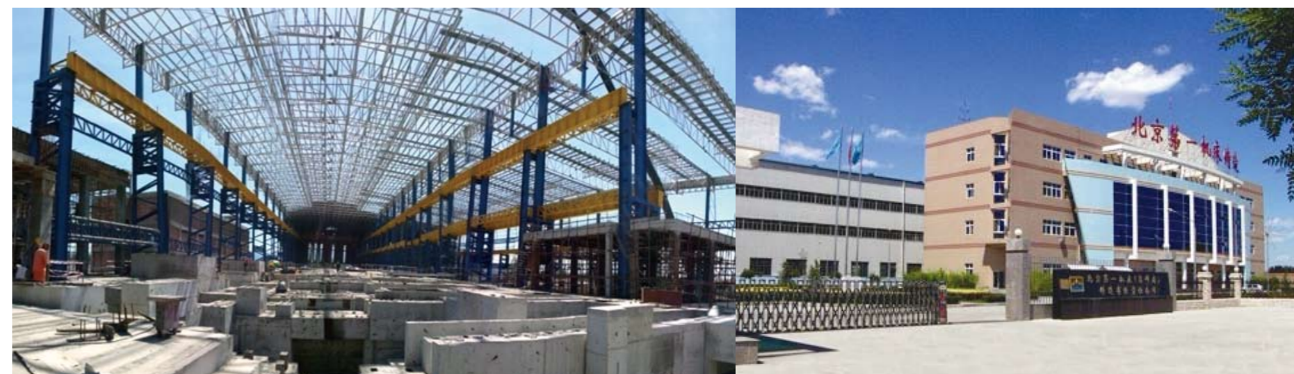
马来西亚槟城钢厂制造与安装项目 Malaysia Penang Steel Plant Manufacture and Installation Project
