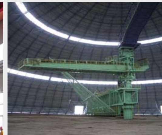
堆取料机 Stacker and reclaimer
