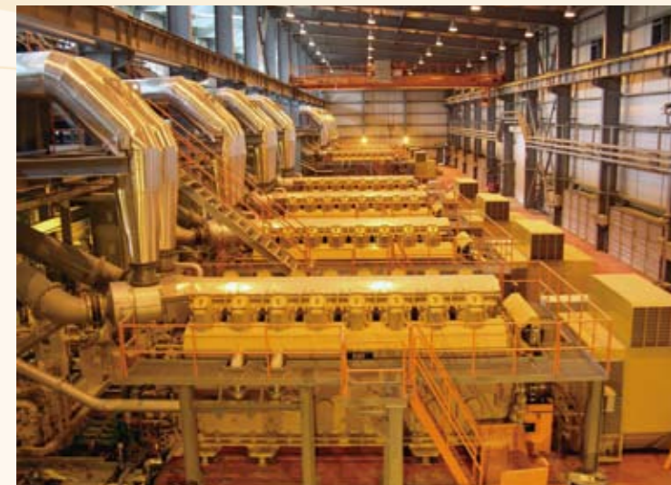
沙特SPCC重油发电厂 Saudi Arabia SPCC Heavy Oil Power Plant
