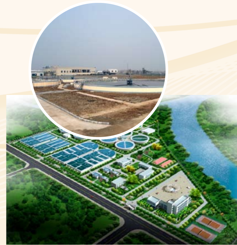
湖北随州污水处理厂二期项目工程 Hubei Suizhou Wastewater Treatment Plant Project (Phase II)
